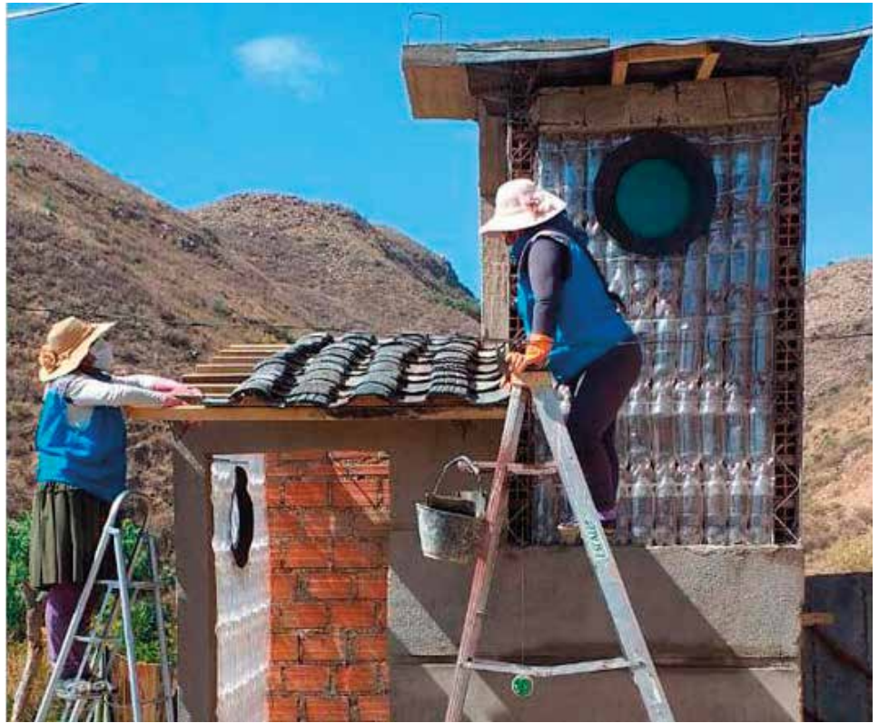
Figure 1. Construction of the sanitary facility. Source: Selavip.org
