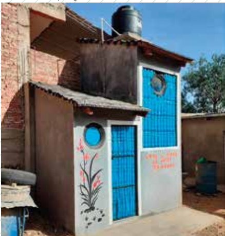
Figure 9. Finished sanitary facility. Source: Hábitat para la Humanidad Bolivia, 2021
