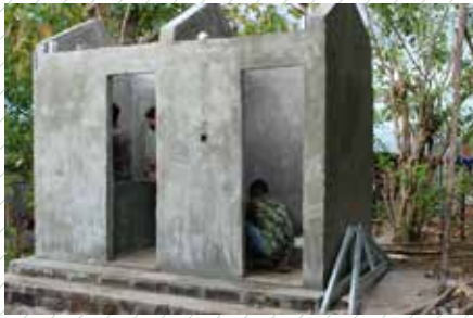
Figure 5. Construction of walls Source: CIRMA, 2020.
