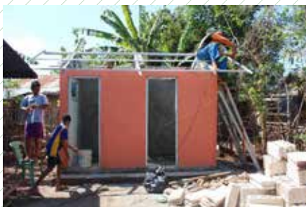
Figure 7. Galvanized canal C assembly. Source: CIRMA, 2020.
