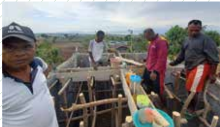
Figure 6. Beam construction. Source: CIRMA-Centrum Inisiatif Rakyat Mandiri Facebook, 2020.
