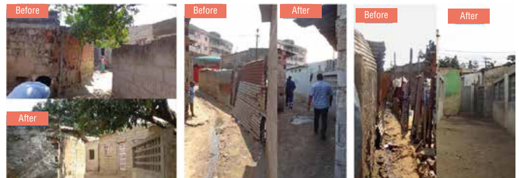
Figure 11. Road widening, before and after. Source: Arquitectos sin Fronteras
